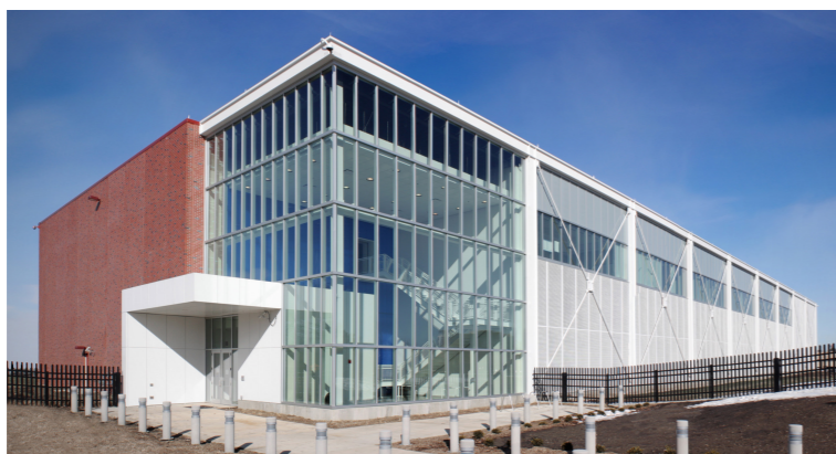
Illinois Petascale Computing Facility
